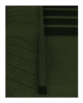
In the case below the developer wished to save time and money by omitting the pin kerb between the ramped access and the car parking bay.
